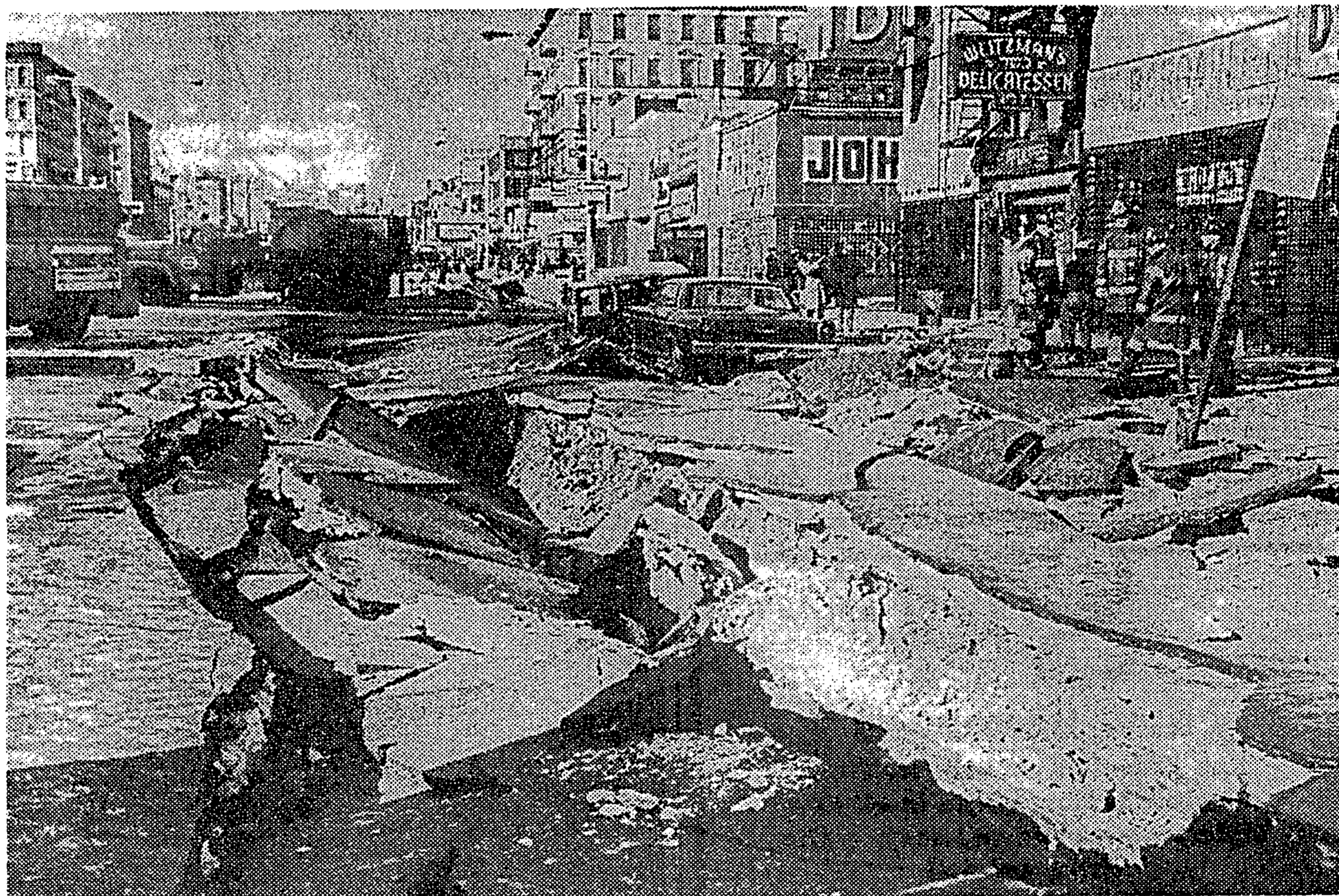
The New York Times (by Robert Walker) SCENE OF GAS EXPLOSION: Ruptured concrete and damaged cars on Delancey Street at Essex Street mark the site where blast occurred Friday night. Many residents of the Lower East Side neighborhood were deprived of heat.
